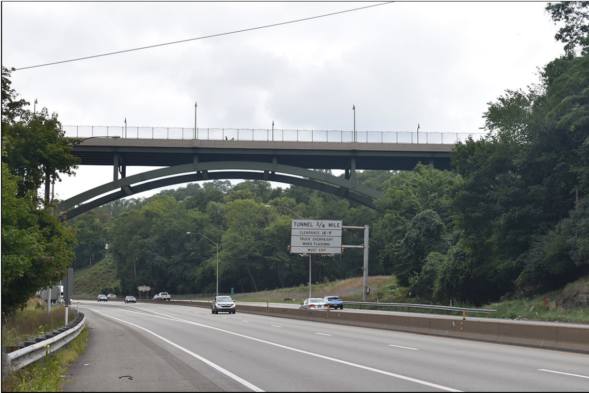
Photograph 23: View looking southeast along I-376 toward the Greenfield Road Bridge.
