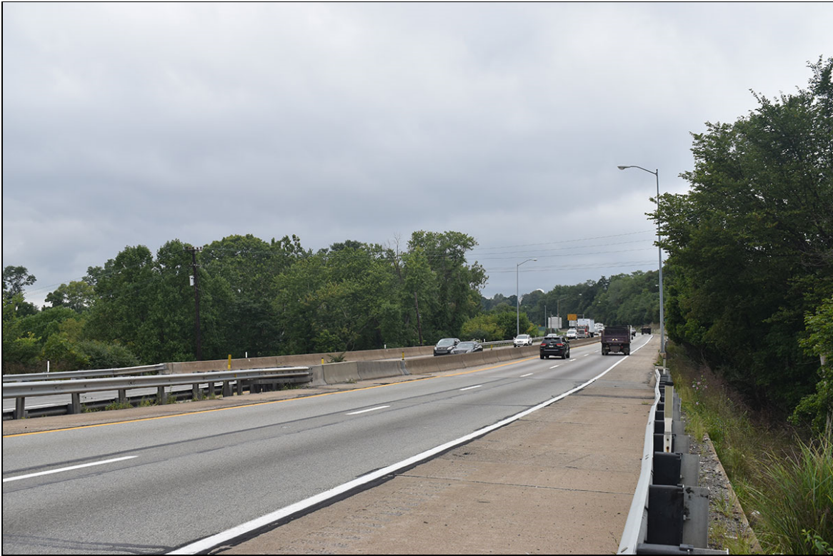
Photograph 3: View looking southwest along I-376 toward the SR 130 overpass.
