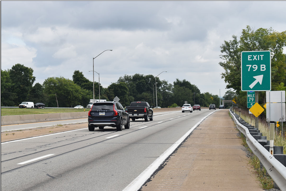
Photograph 2: View looking east along I-376, near Exit 79B.
