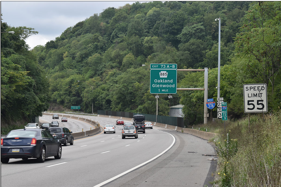
Photograph 24: View looking west along I-376.
