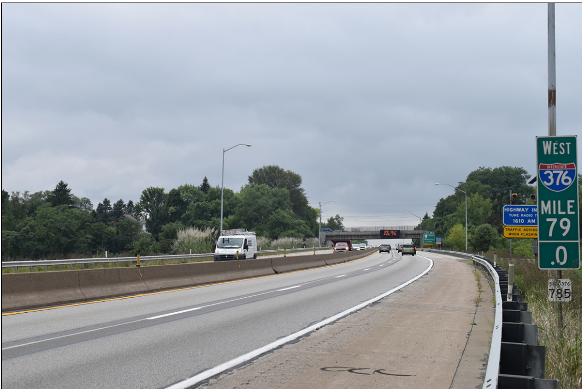
Photograph 4: View looking southwest along I-376.
