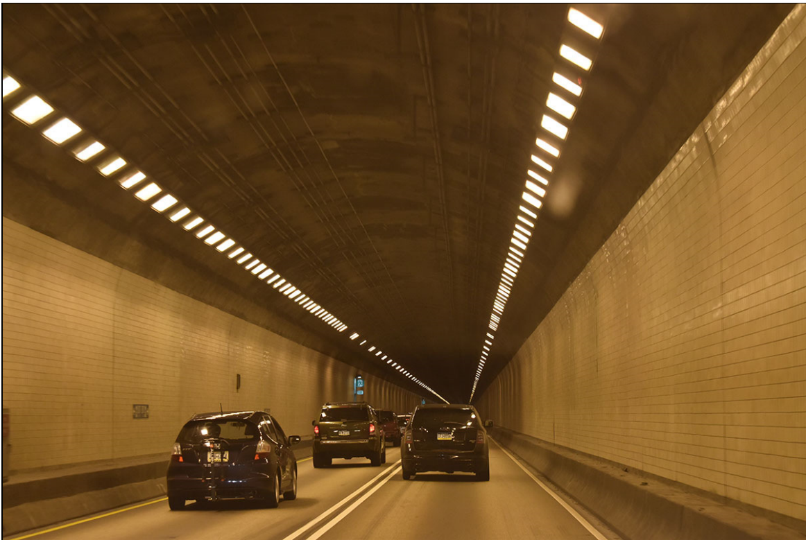
Photograph 20: View of the interior of the Squirrel Hill Tunnel, a contributing element of the Penn-Lincoln Parkway East.
