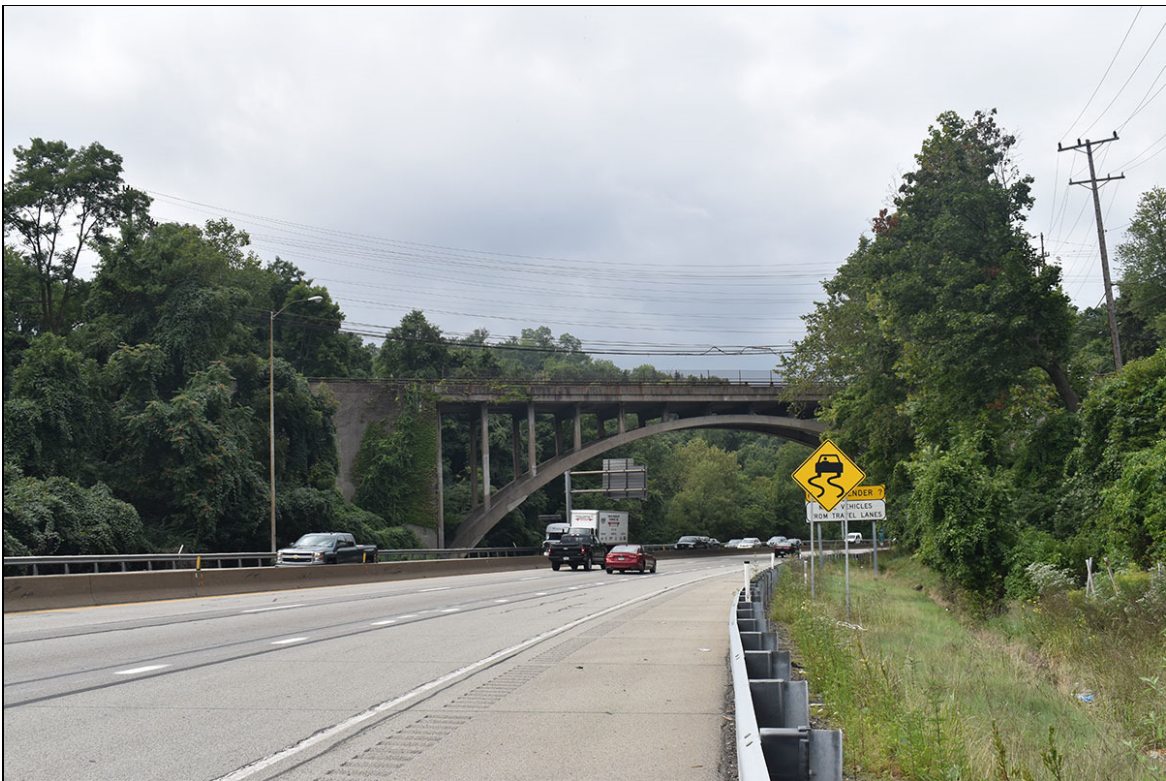
Photograph 10: View looking southwest along I-376 toward the Maple Avenue Bridge.
