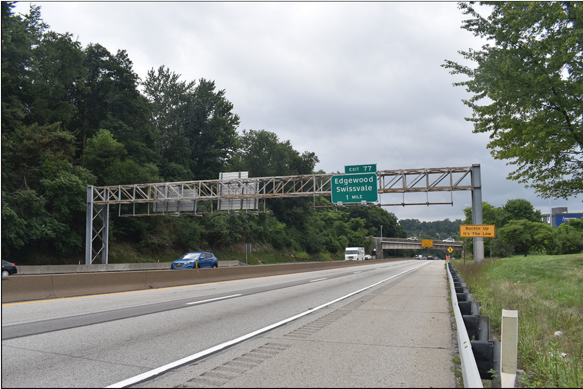
Photograph 8: View looking southwest along I-376 near the Edgewood/Swissvale exit.
