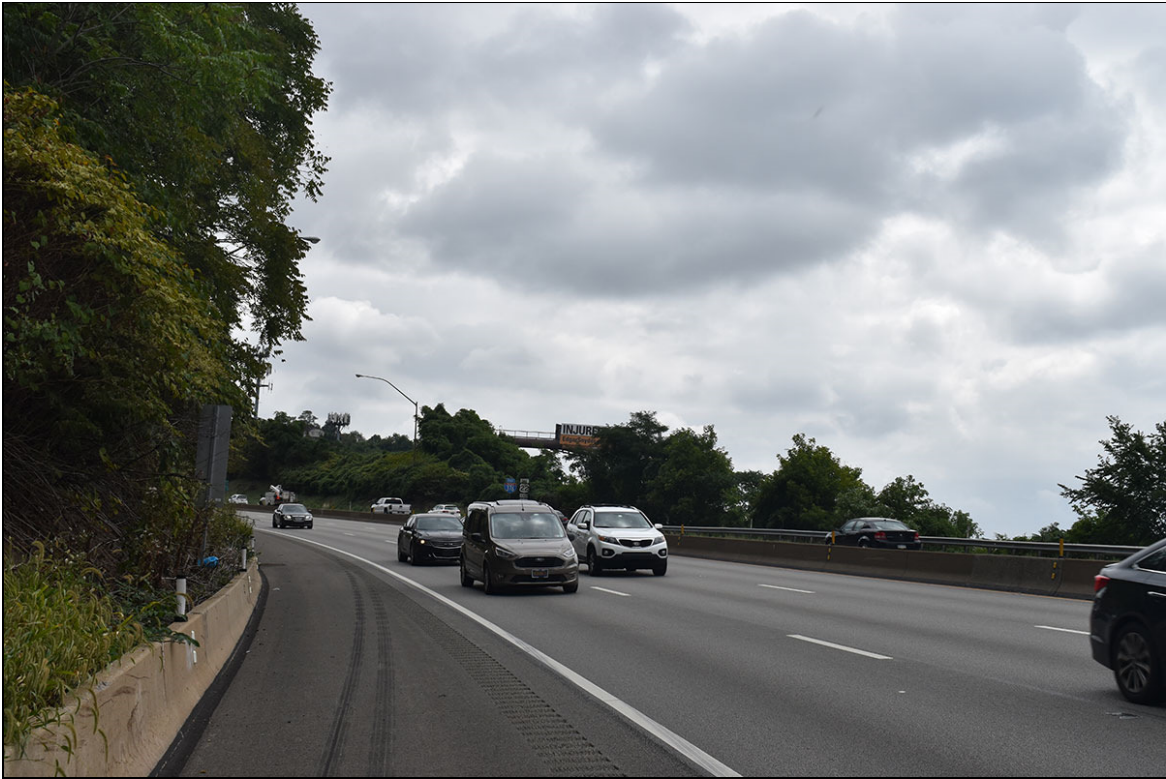
Photograph 29: View looking southeast along I-376.
