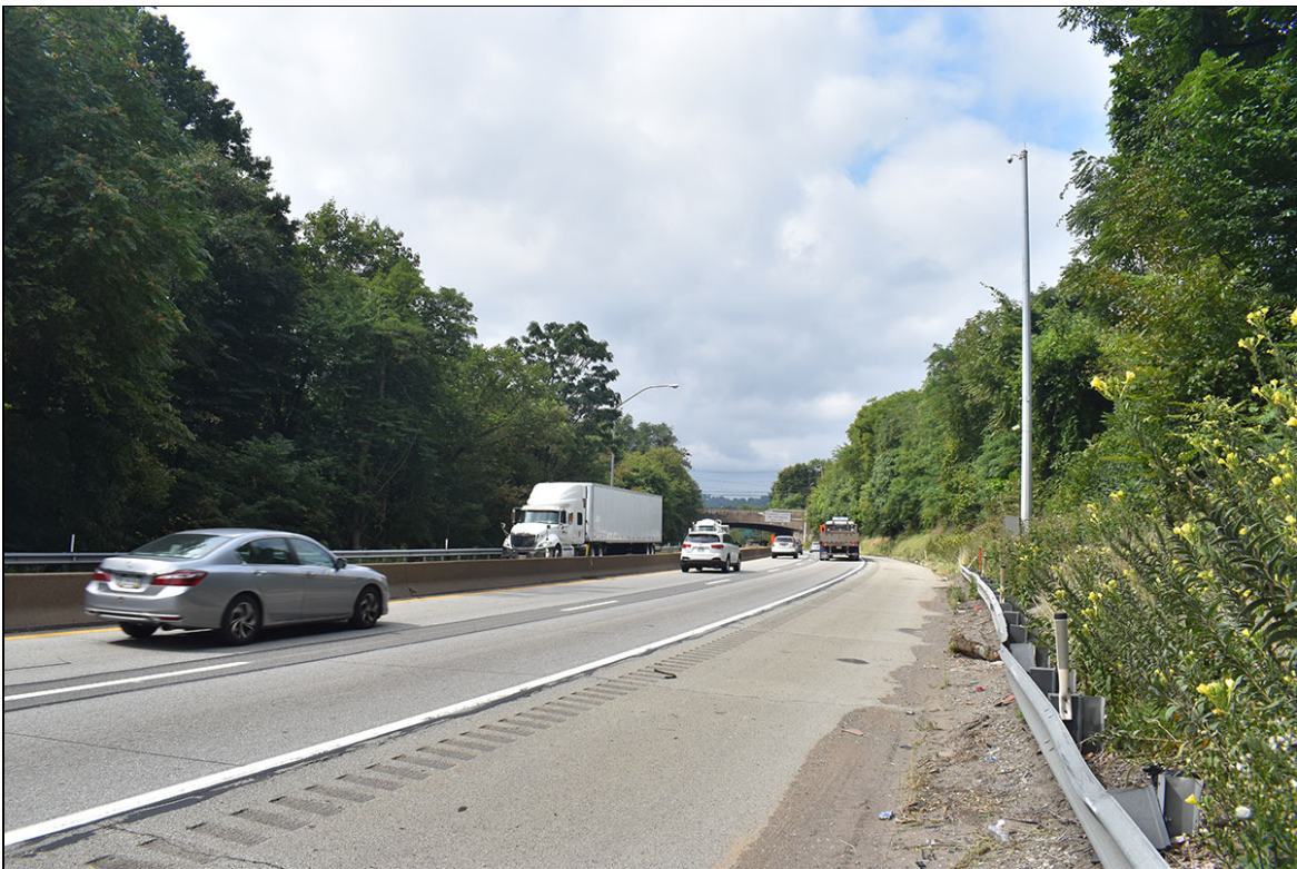
Photograph 14: View looking southwest along I-376 in Edgewood Borough.
