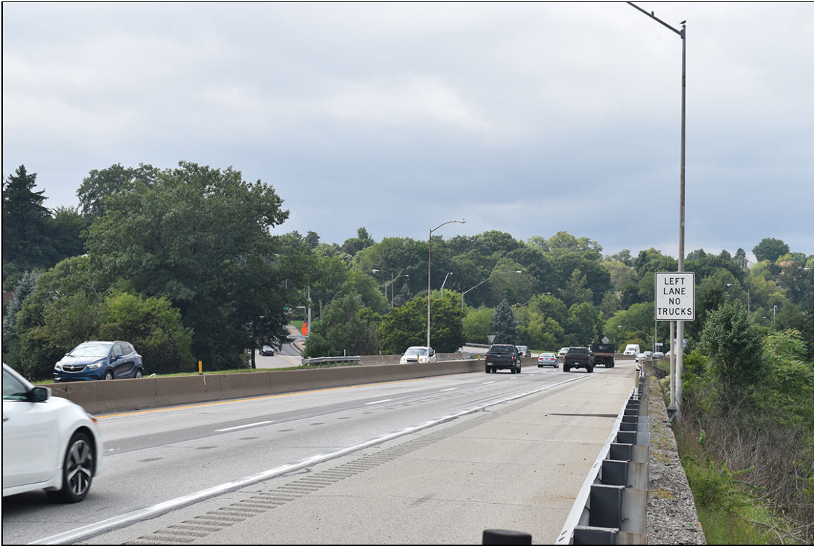
Photograph 17: View looking southwest along I-376 toward the bridge over S. Braddock Avenue.
