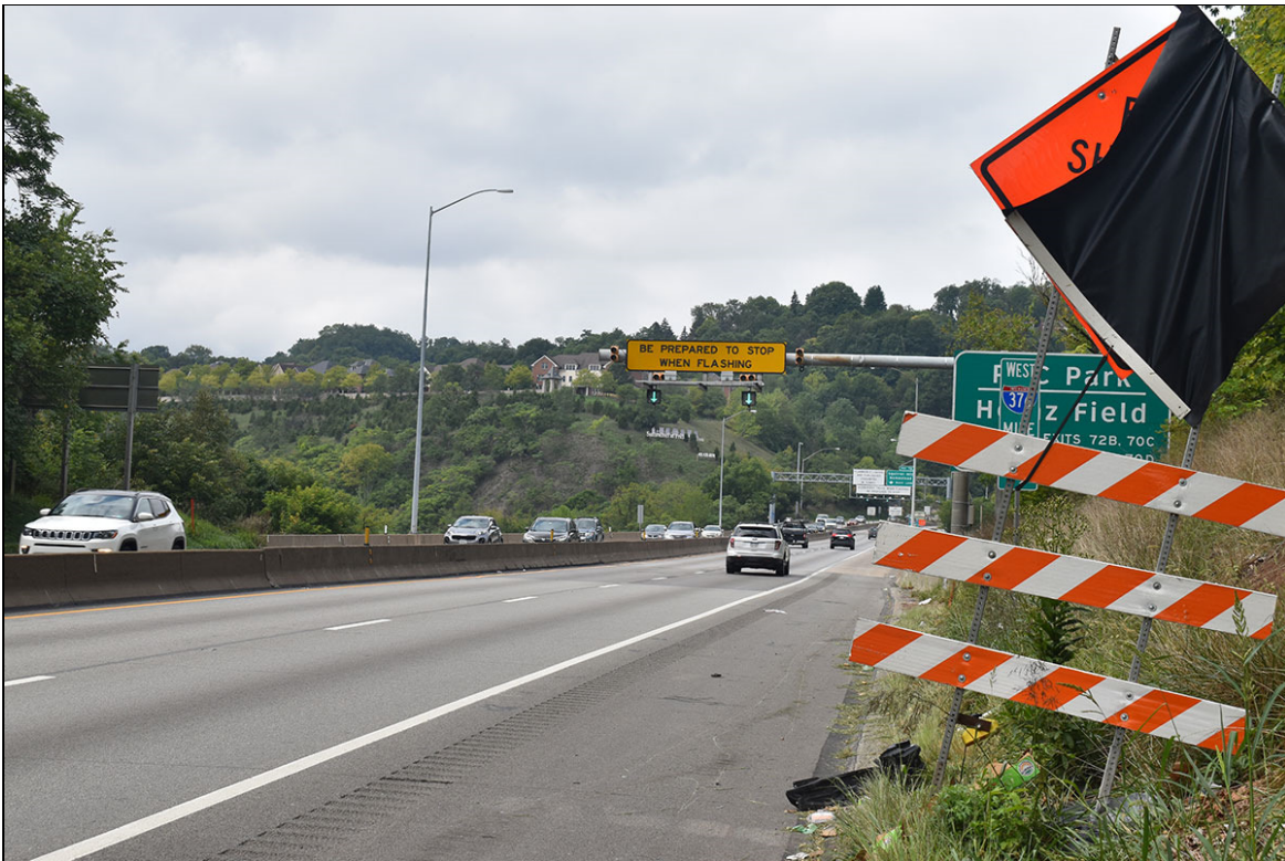
Photograph 18: View looking west along I-376 toward the bridge over Commercial Street.
