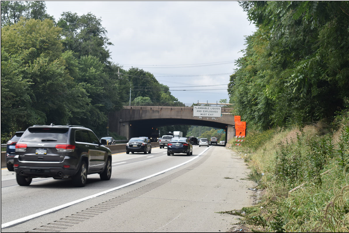
Photograph 15: View looking southwest along I-376 toward the Edgewood Avenue Bridge.
