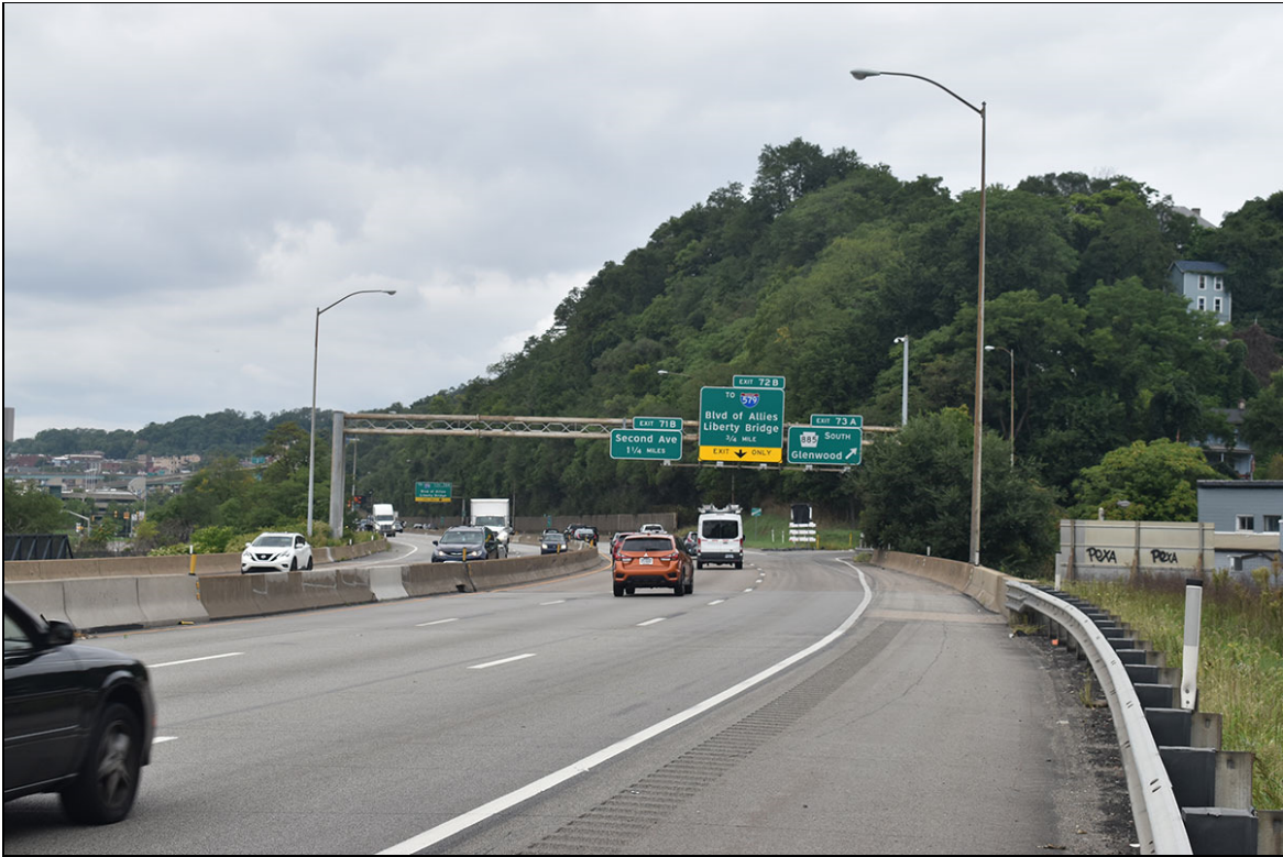
Photograph 31: View looking northwest along I-376 toward the Bates Street Interchange.
