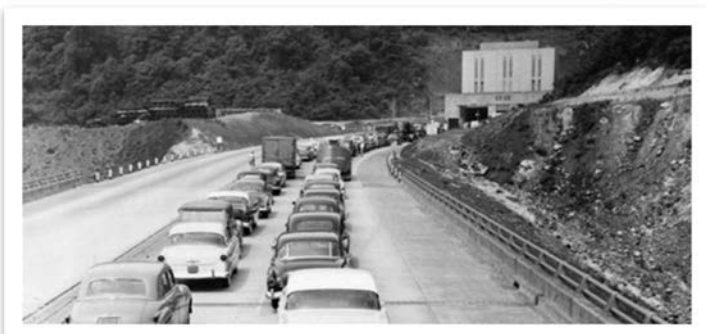
Traffic approaches Squirrel Hill Tunnel c. 1960.
