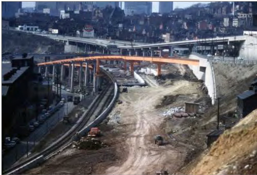
Figure 14: Parkway East Construction in the late 1950s.
