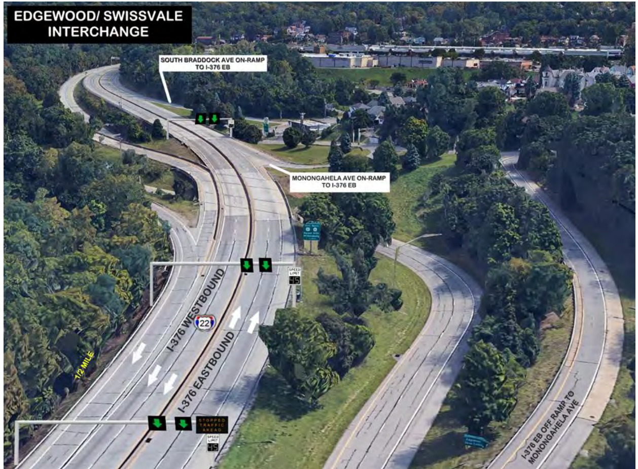
Figure 31: Example of Additional Dynamic Messaging Signs
