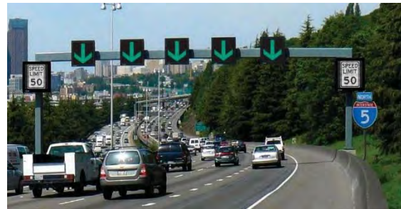
Figure 4: Example of Dynamic Lane Use Control. Photo and Illustration. Example of full gantry ATM deployment in Washington State (Source: WSDOT).
