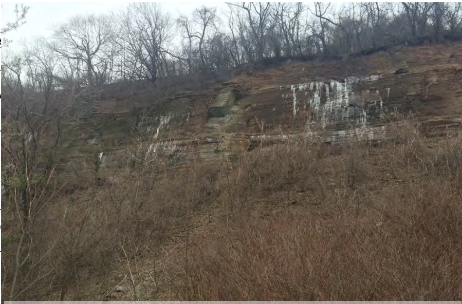
UNDERCUT ROCKBLOCK NEAR TOP OF SLOPE ILLUSTRATES VALLEY STRESS AND TECTONIC JOINT SETS.
