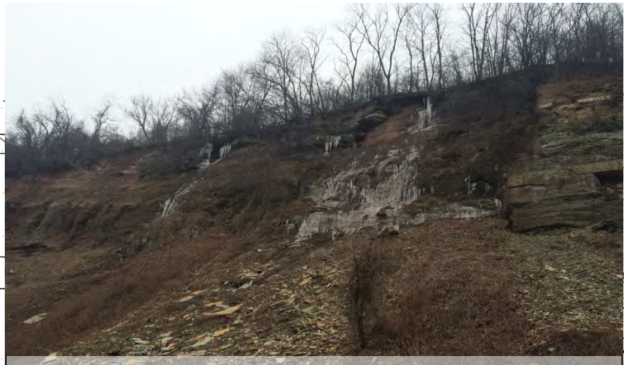
ROCKFALL FROM TOP OF SLOPE. DEBRIS PATH EXTENDS TO EDGE OF BUSWAY. LARGE OVERHANGS POSE ADDITIONAL ROCKFALL THREAT TO BUSWAY. RECOMMEND REMOVAL OF ROCKFALL DEBRIS FROM CATCHMENT AREA BETWEEN STA. 230+00 AND 237+00.
