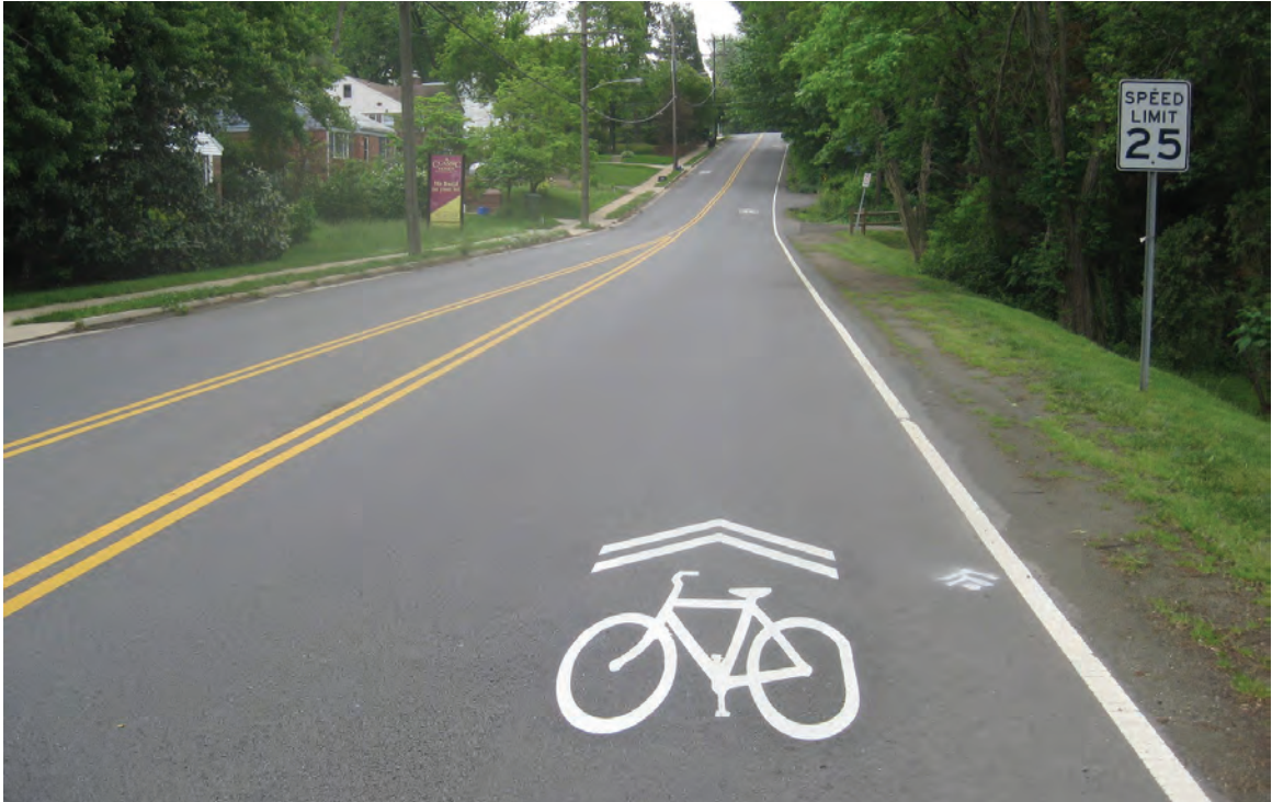
Shared Lane Marking
