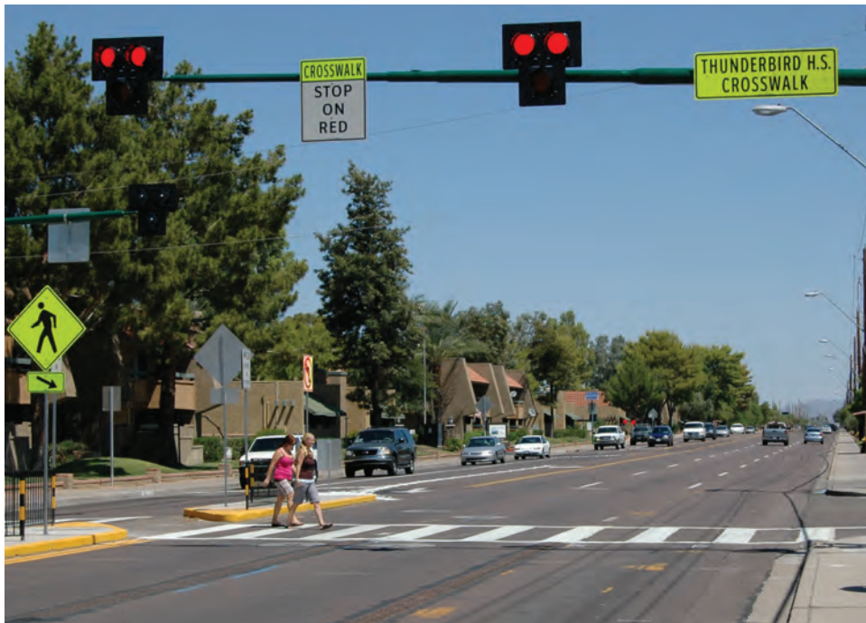
Overhead Signs and Flashing Beacons
