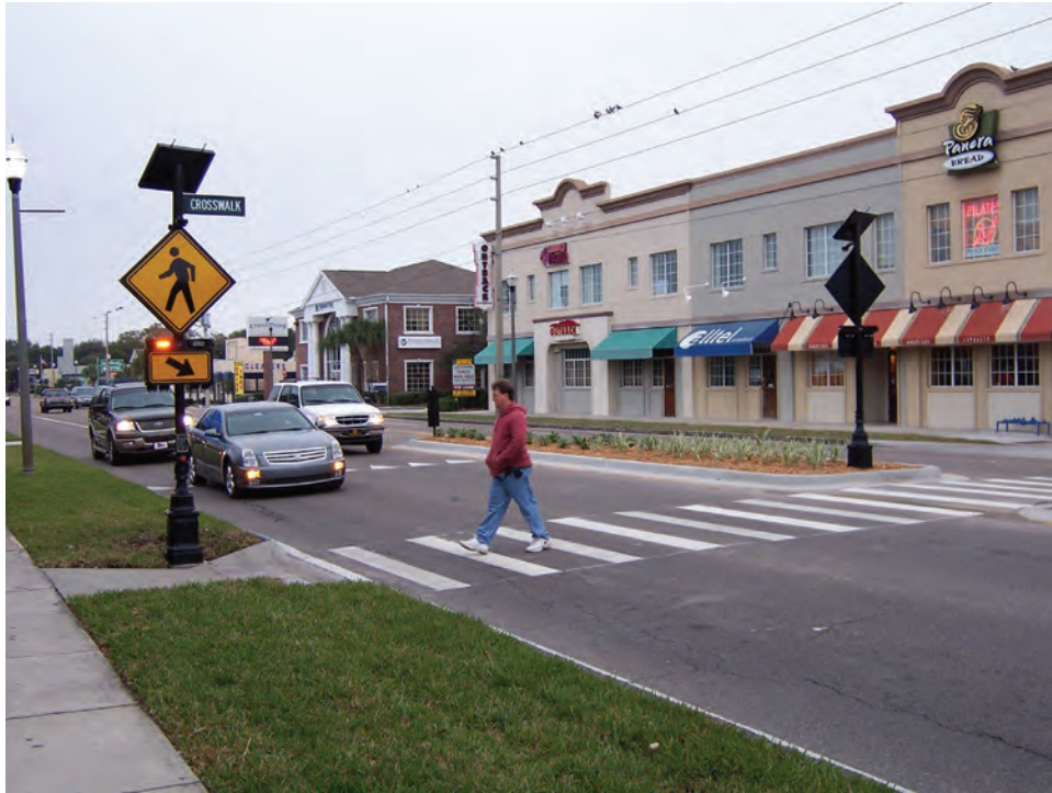
Pedestrian Warning signs
