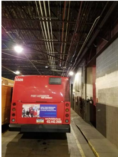
Figure 33 Egress Aisle at Wall
