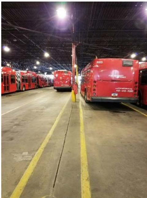
Figure 31 Aisle at Structural Columns
