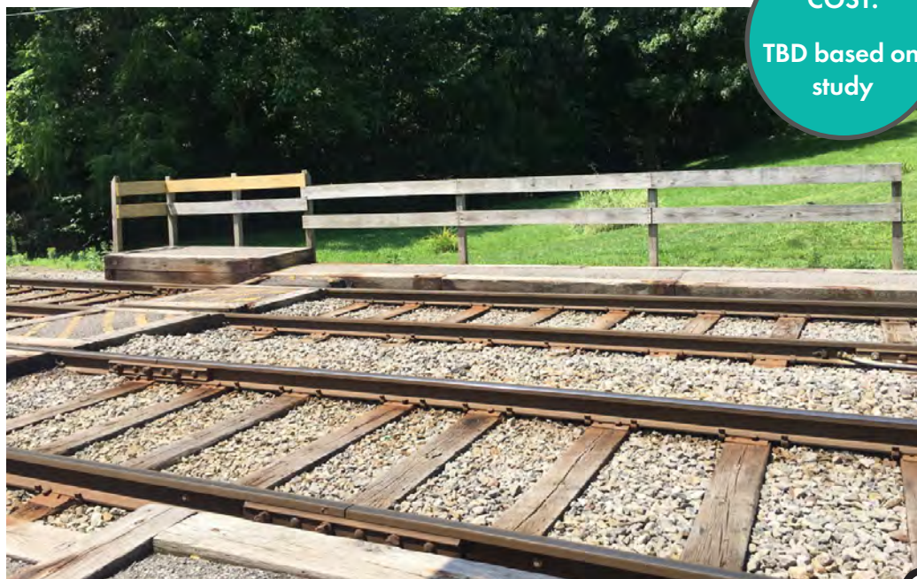
Existing conditions at Hillcrest Station, Library Line, Bethel Park
