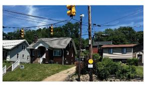
This project added new controller assemblies, emergency vehicle preemption (EVP), replaced electrical services, and faded pavement markings. Additionally, this project added GPS units in conjunction with new coordinated timing plans to provide coordination and maintain traffic flow.
