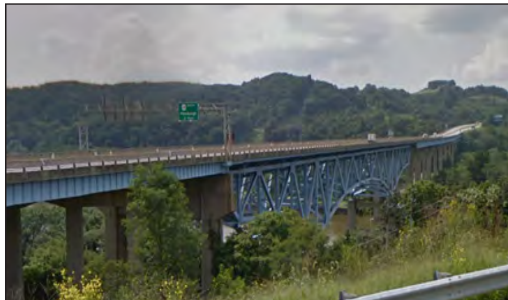
Judge J. Franklin Graff Bridge in North Buffalo and Manor Townships
