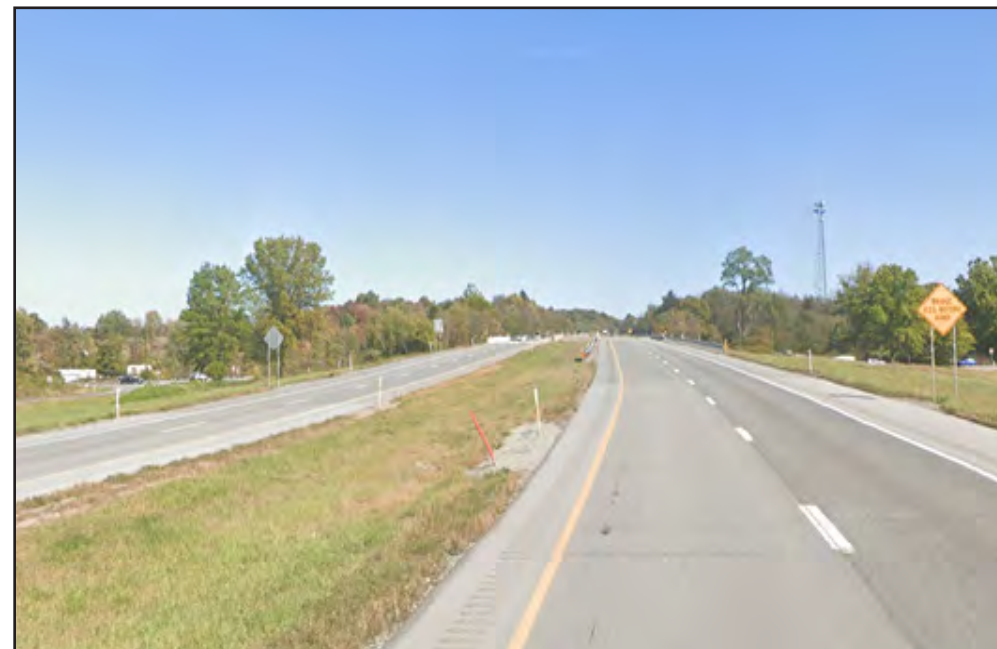
Looking East, US 422 at SR 954 in White Township
