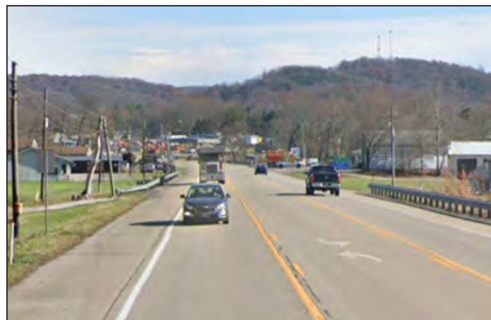
Looking East, US 422 through Shelocta Borough
