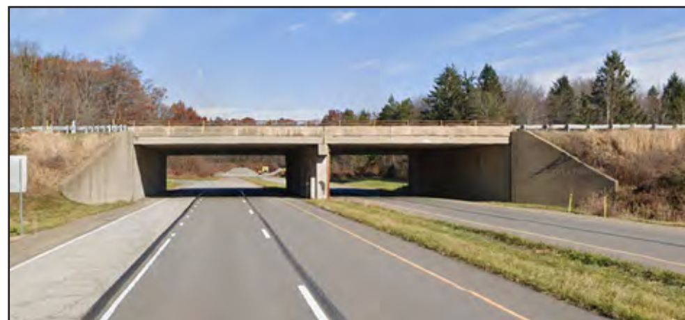
US 422 Bridge over SR 356 in Butler Township
