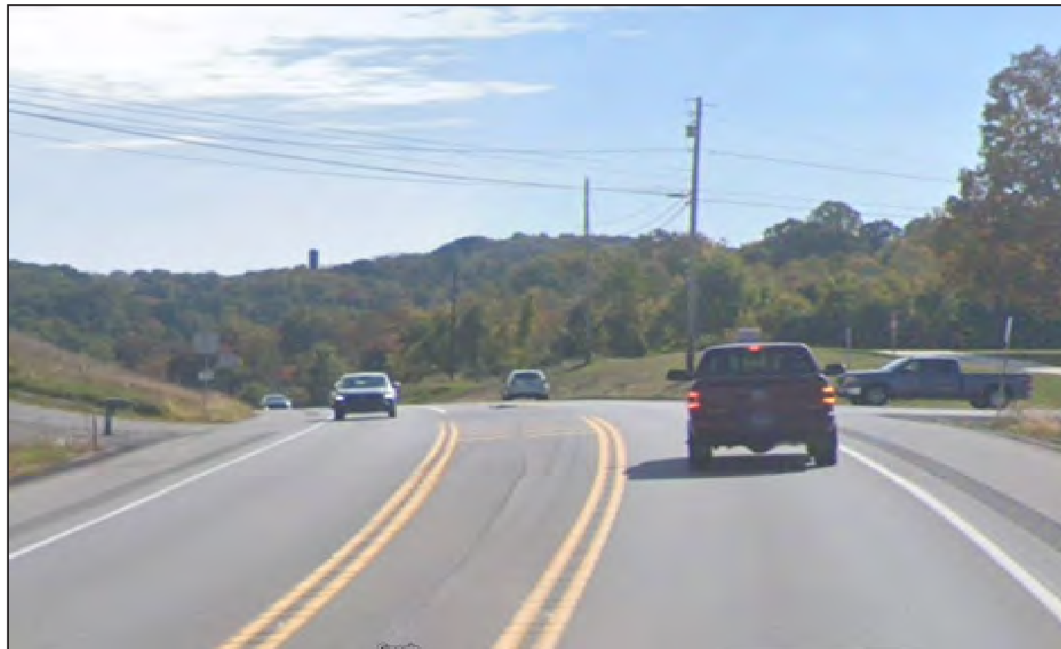
US 422 at Silvis Hollow Road in Kittanning Township 92
