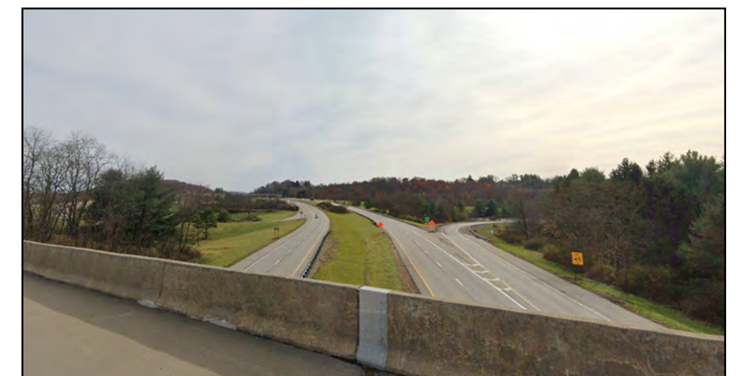
Looking East, US 422 at the Business 422/SR 268 in East Franklin Township
