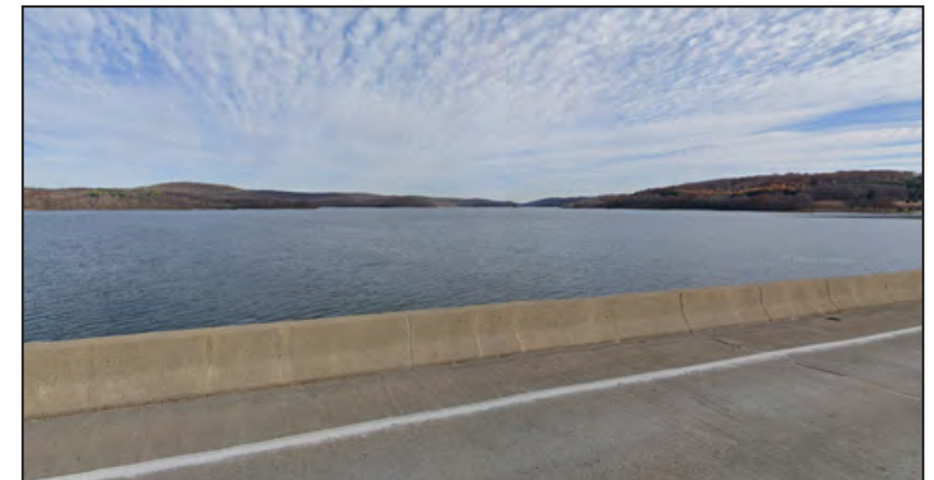
US 422 Bridge over Lake Arthur
