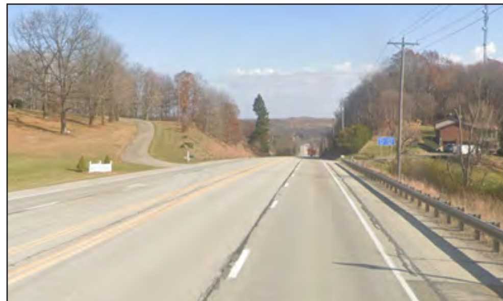
Looking East, US 422 at the Butler/Armstrong County Line
