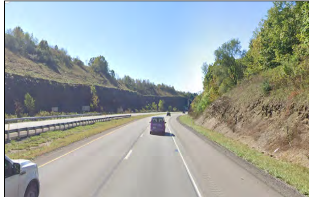
Looking West: US 422, Kittanning Bypass, between SR 28 and the Kittanning/SR 66 interchange in Manor Township
