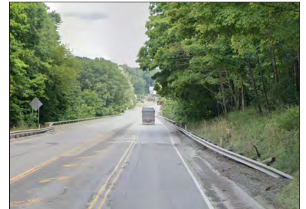
US 422 over Slippery Rock Creek in Slippery Rock Township
