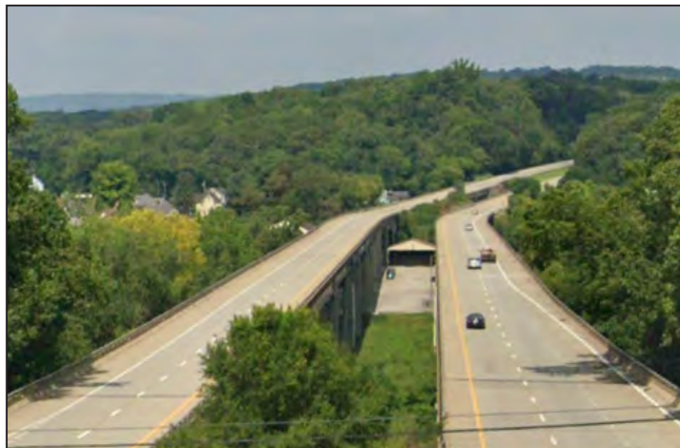
US 422 over the Shenango River and SR 18 in Taylor, Union, Mahoning Townships and the City of New Castle
