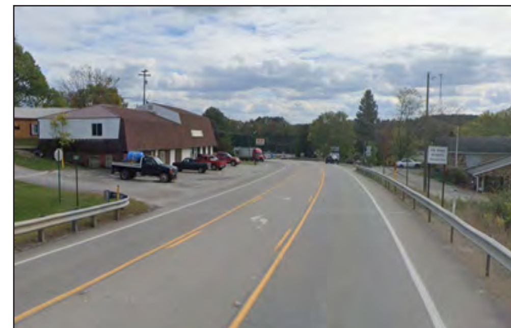
Looking East, US 422 in Elderton Borough
