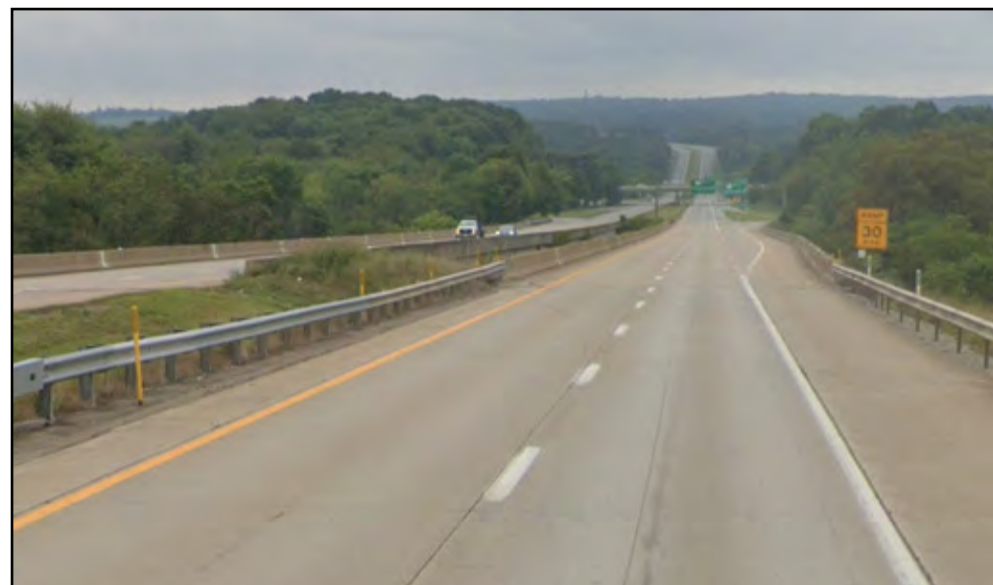
Bridge to Nowhere, US 422 over SR 4422 (Ben Franklin Road), SR 4005 (Indian Springs Rd), SR 3035 (Old US 119), and the Buffalo and Pittsburgh Railroad in White Township
