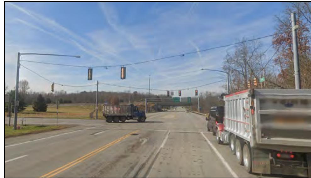
US 422 at Northbound I-79 Ramps in Muddy Creek Township
