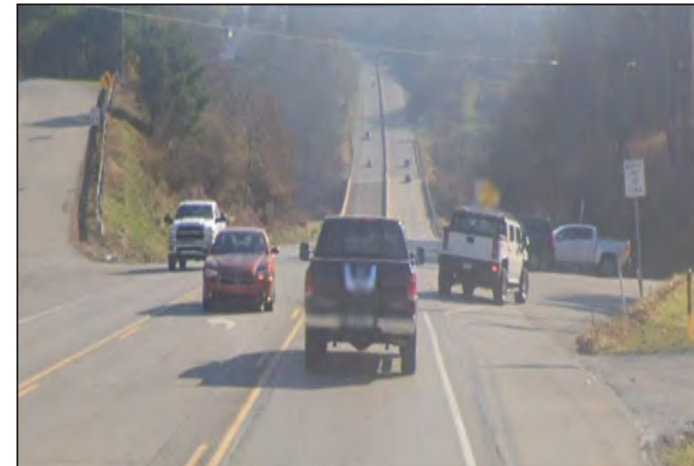
US 422 at Greenwood Road intersection
