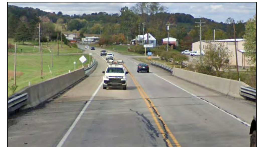
US 422 near Plum Creek, Plumcreek Township
