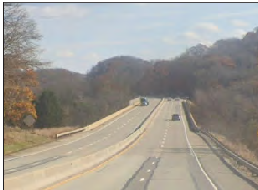
Looking East: Worthington No. 1 Bridge, US 422 over Buffalo Creek
