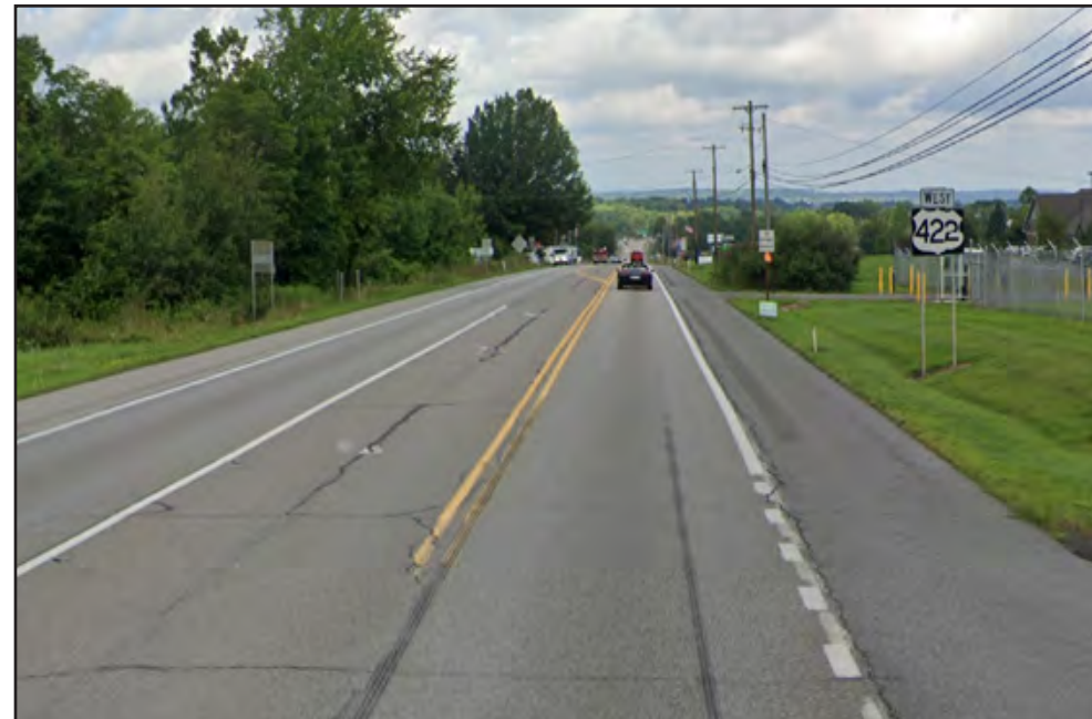
US 422 looking west towards New Butler Road Intersection in Shenango Township
