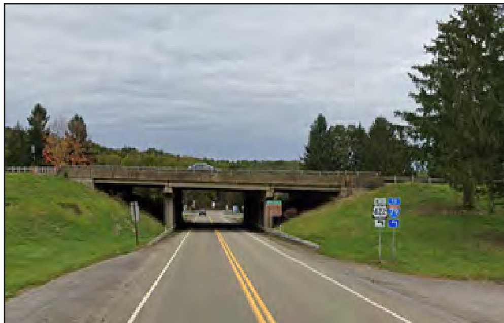
US 422 Bridges over SR 4005 (Pleasant Valley Road) in Muddy Creek Township
